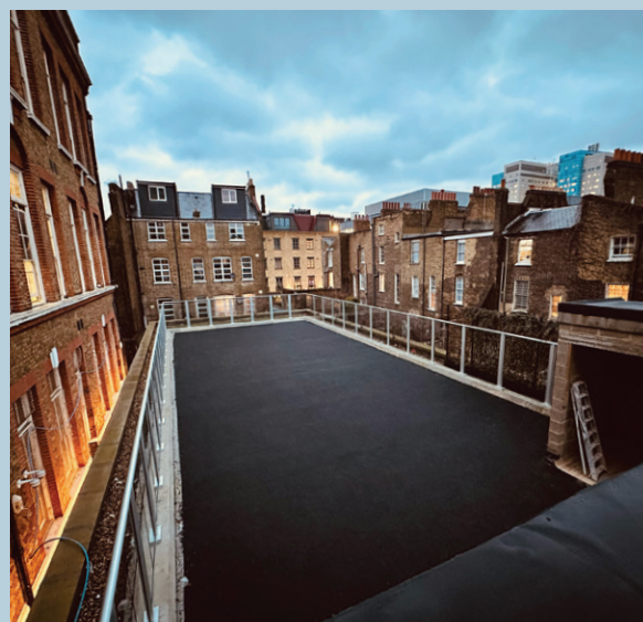
Blue Roof project at Madani Girls' School
