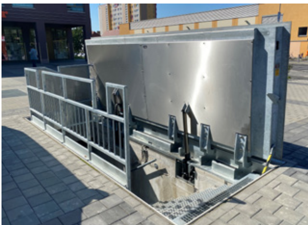
Hydraulic escape hatch with collapse protection, Berlin
