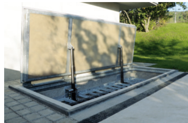
Hydraulic cover on a woodchip silo with a fire protection classification of F90, Eisenstadt/Austria
