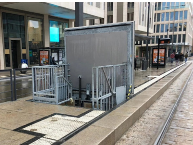
Truck-accessible, watertight, hydraulic transformer covers with thermal insulation, Luxembourg
