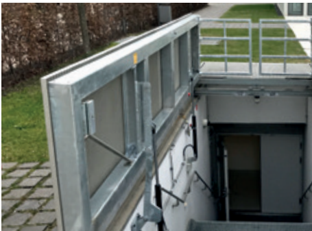
Large, rectangular covers on structural openings
