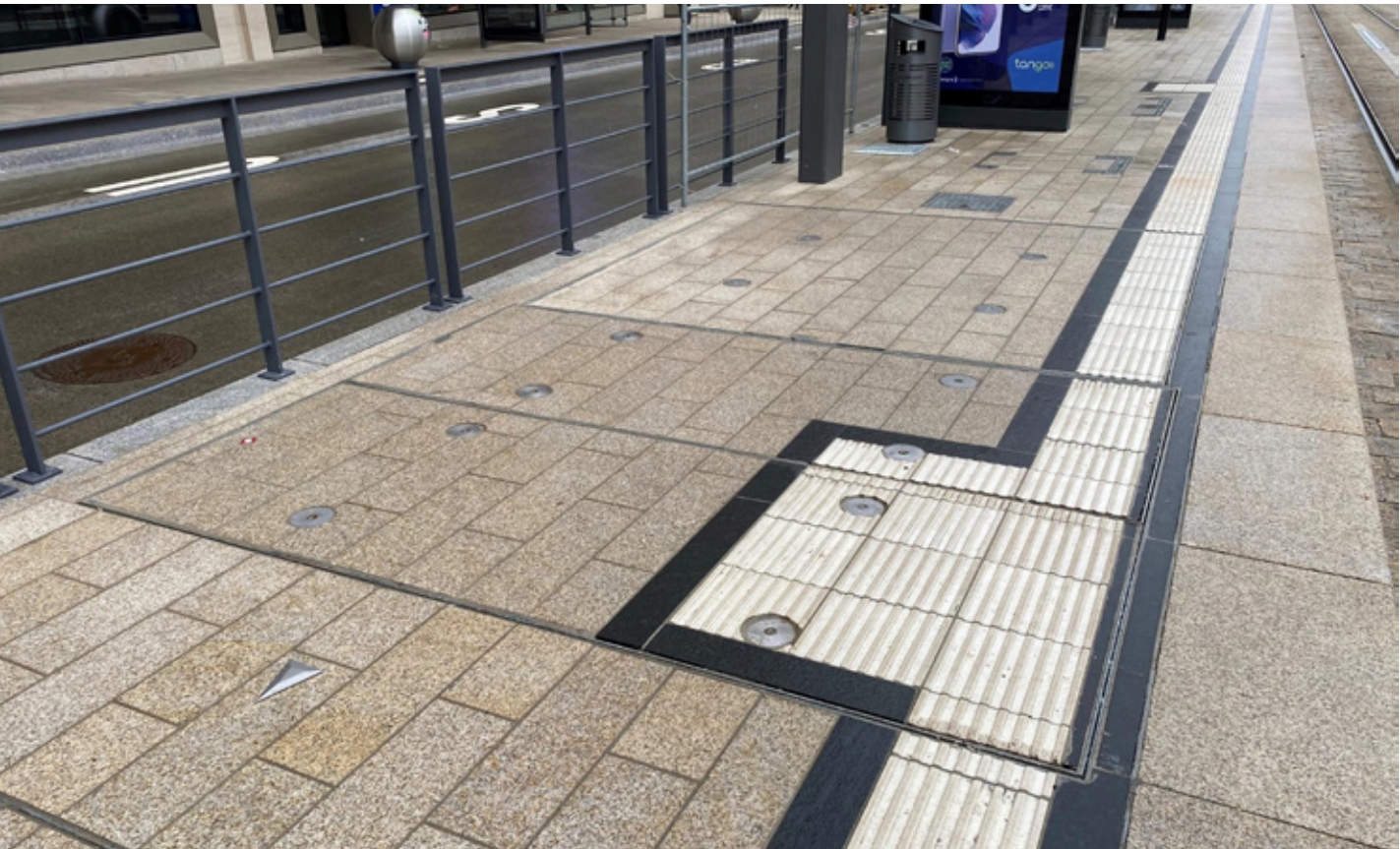
Discreet, as little metal on the surface as possible – this can be realised with pavalable floor hatches, Luxembourg
