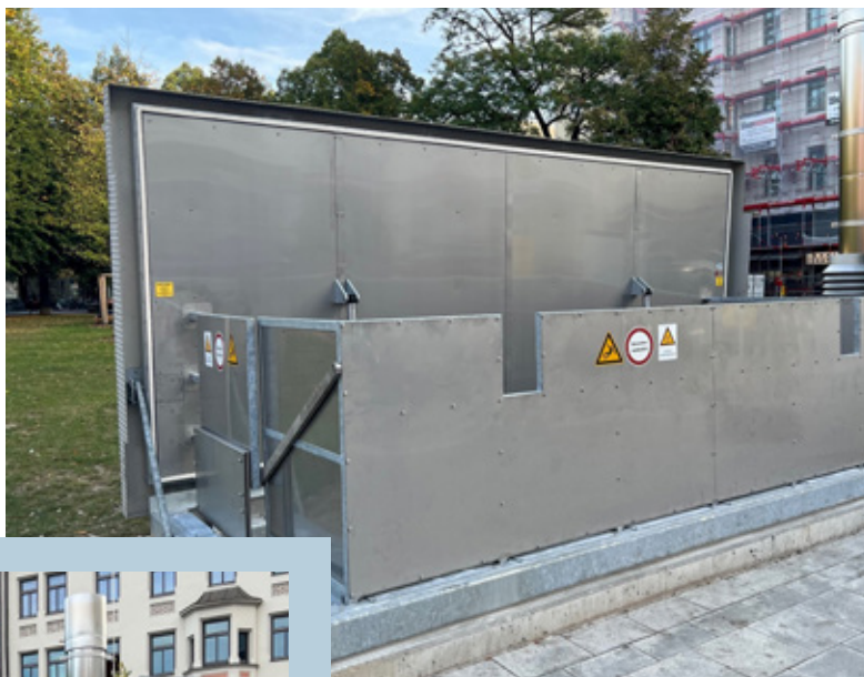
Hydraulically actuated smoke extraction damper with collapse protection at the Isartor, Munich
