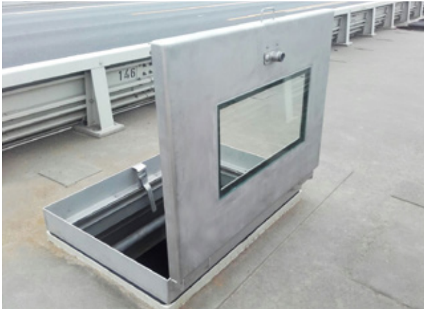
Small escape hatch that can be opened by hand
