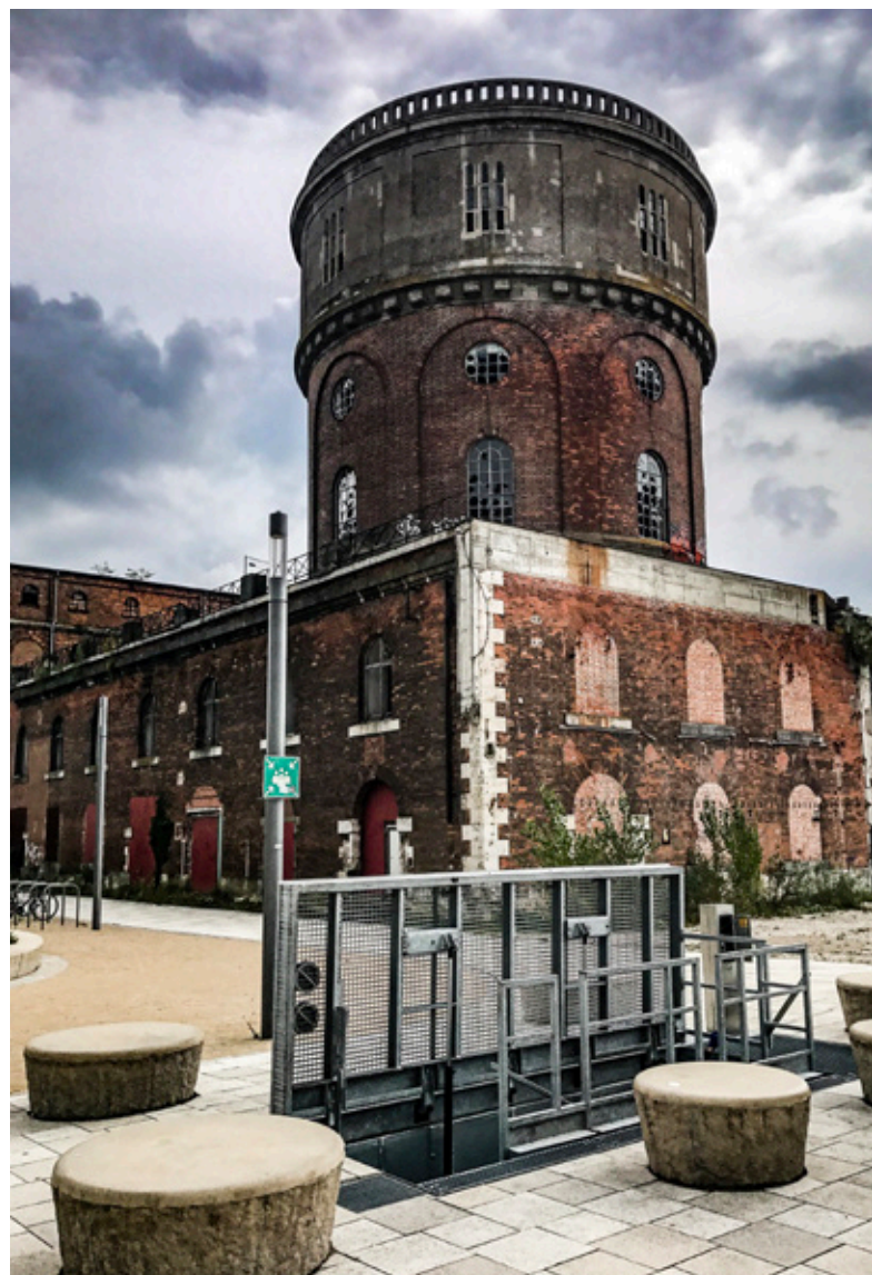
Escape hatch with a hydraulic drive and grating, Ingolstadt
