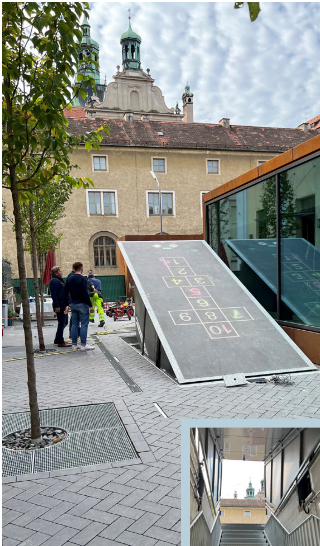
Automatic opening even in the event of a power failure thanks to hydraulic pressure accumulators with integrated emergency power supply, Munich State Archaeological Collection
