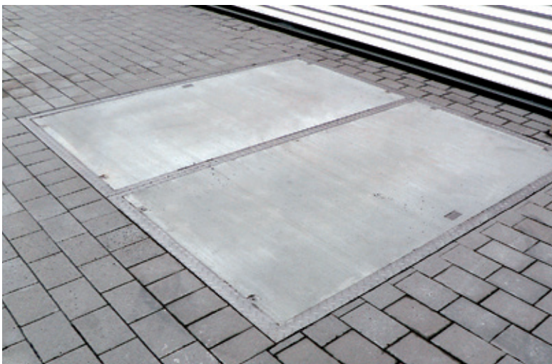
Two-piece shaft cover with concrete surface, Frankfurt
