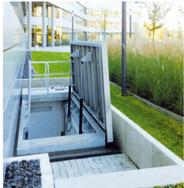
Hydraulic stainless steel escape hatch, Cologne
