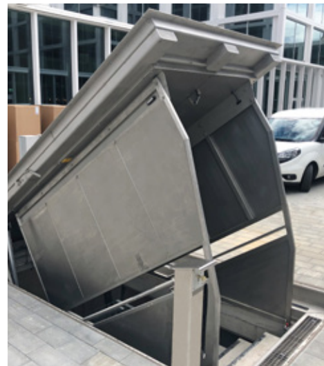
Hydraulic escape hatch cover, Stuttgart
