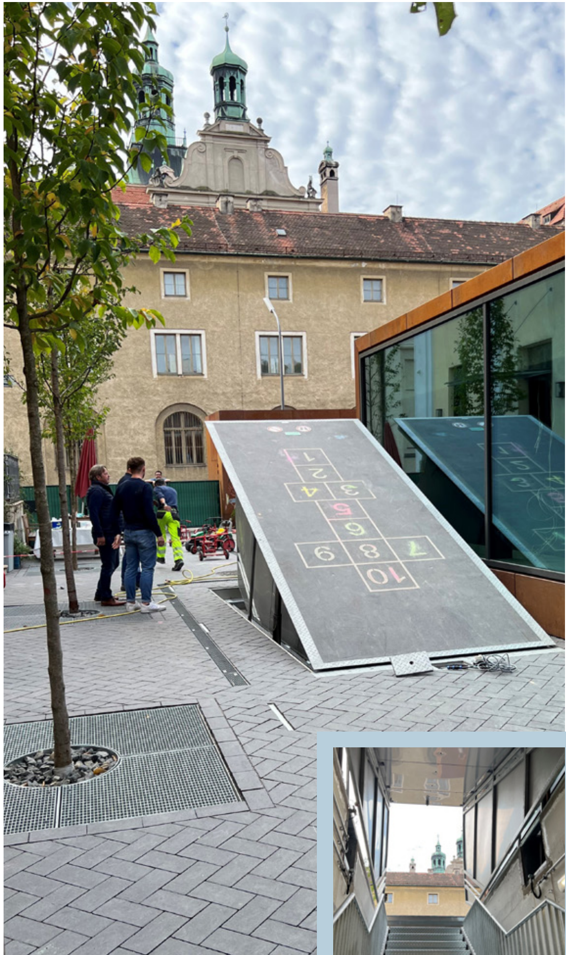
Automatic opening even in the event of a power failure thanks to hydraulic pressure accumulators with integrated emergency power supply, Munich State Archaeological Collection
