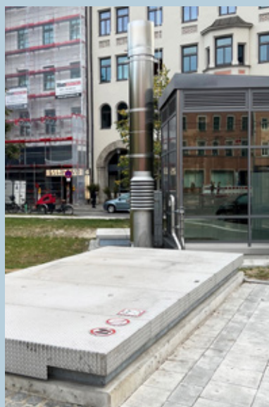
Hydraulically actuated smoke extraction damper with collapse protection at the Isartor, Munich
