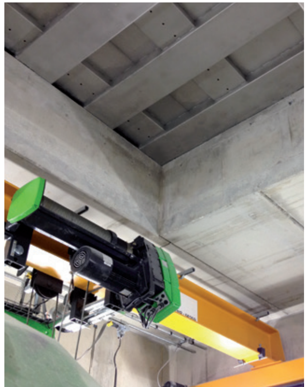
View from below of a floodproof cover on an assembly opening, power plant on the river Danube near Augsburg
