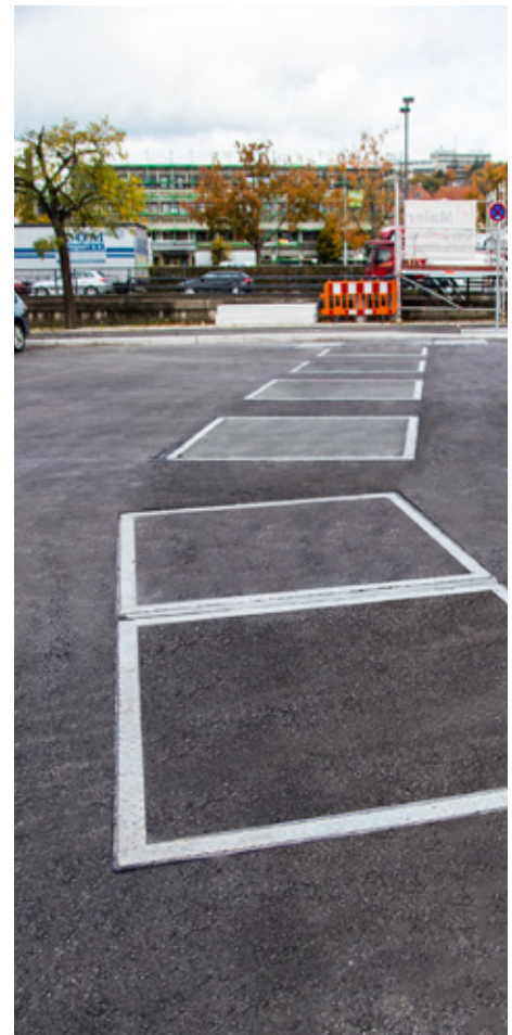
Backwater-proof covers filled with asphalt, Ansbach
