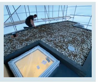
A successful blue roof retrofit project was carried out on an extended building in central London, using ACO Building Drainage's innovative RoofBloxx attenuation system. This project presented significant challenges, particularly in managing water runoff while adhering to sustainable urban drainage system (SuDS) requirements set by The Royal Borough of Kensington and Chelsea (RBKC).
