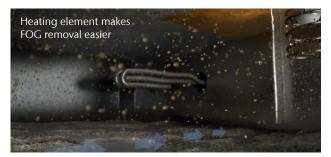
The heating element placed in the FOG layer keeps it liquid making it easier to be removed through the valve arrangements.
