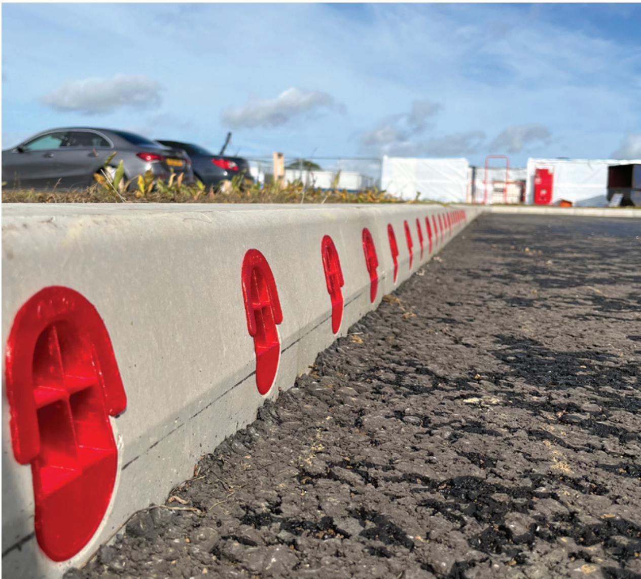
Photo shows Installation prior to completion
