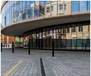
Gary Morton, Head of Stakeholder Engagement at ACO explains, "Around the immediate façade of the Blavatnik building, a thin protective line of ACO MultiDrain MD Brickslot has been installed to collect water before it reaches the building and its entrances.
