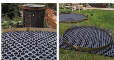
Installation of RoofBloxx Reservoir tray (30mm) to create irrigation for sedum roof in picture above
