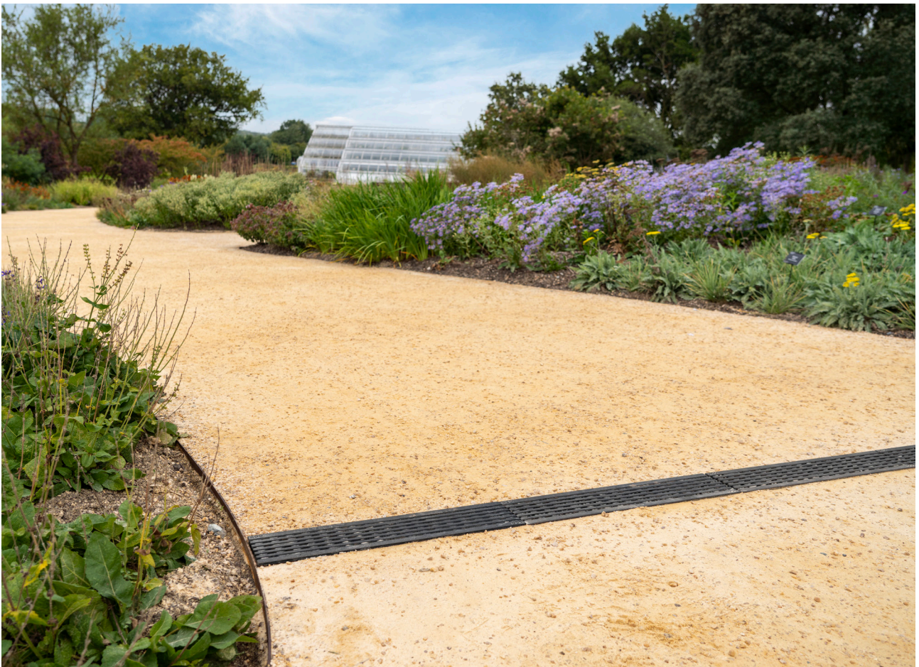
ACO channel drains across the path capture runoff and direct it into soakaways constructed under the planting.
