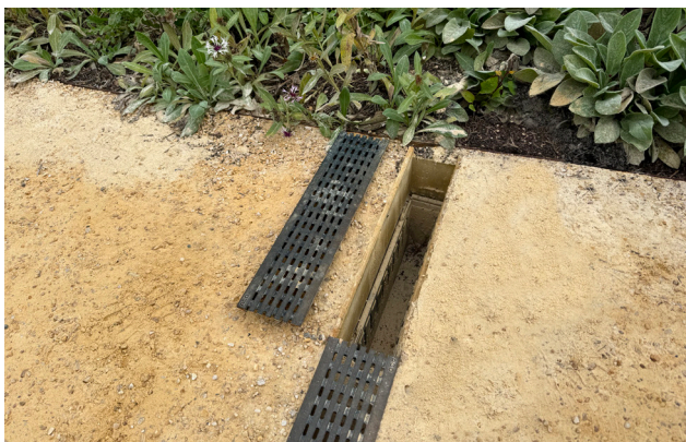
Sump units, installed at each outlet, capture silt and protect soakaway from clogging up.
